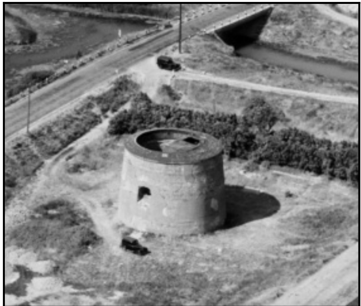
Top photo shows Obs Woodland and Obs Wraight on duty at the M2 Dymchurch Post. Below shows a 1949 photo of Martello Tower No 25. Note what appears to be a WW2 type ROC aircraft reporting post in the top of the tower, including instrument pedestal and flat laying glass panels.
